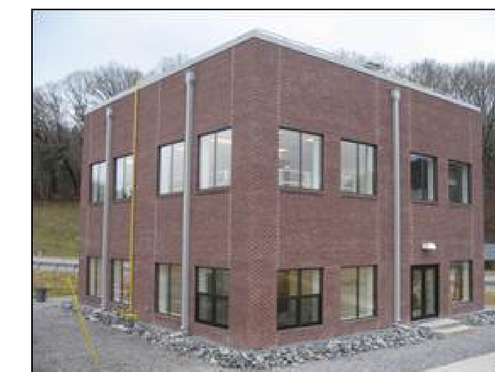
Figure 3. Physical two story FRP structure – located near MAXLAB.
