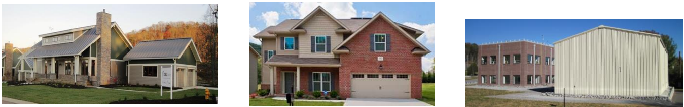
Figure 1 These are photos of ZEBRAlliance House 1 at the left (Miller et al. 2012), a home at Campbell Creek in the middle (TVA. 2010), and the 1-story and 2-story Flexible Research Platforms that represent light commercial buildings at Oak Ridge National Laboratory shown to the right (Hughes. 2012).
