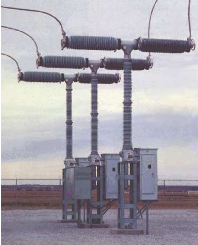
Live-tank breakers
