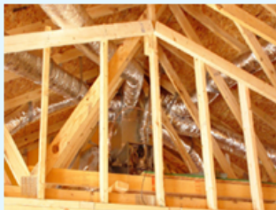
Ducts in the Attic
