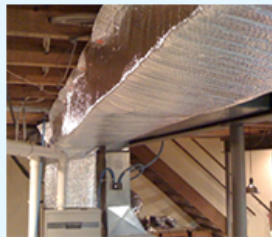
Ducts in a Conditioned Space
