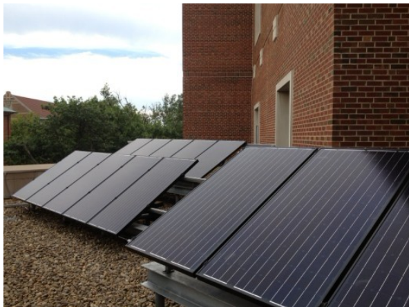
(a) Solar panels Astronergy CHSM-5612M
