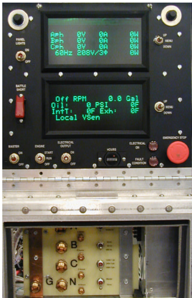
Fig.13. Gen-set user interface and display panel (top half of picture) and field output connections and voltage configuration and frequency selection switches (bottom half of picture).
