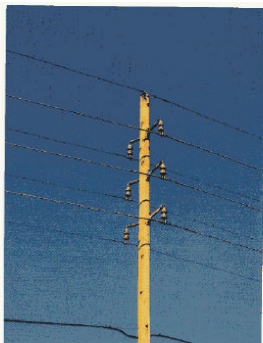
Fig. 3. An example of lightning-resistant construction techniques with two 3-phase feeders on one pole.
