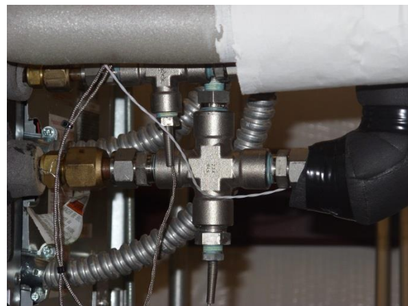
Refrigerant Temp and Press
