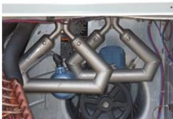
Refrigerant mass flow
