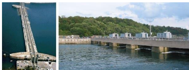
Figure 6. Rance Tidal Power Station
