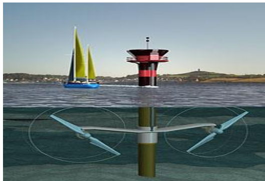
Figure 2. SeaGen Tidal Stream Generator
