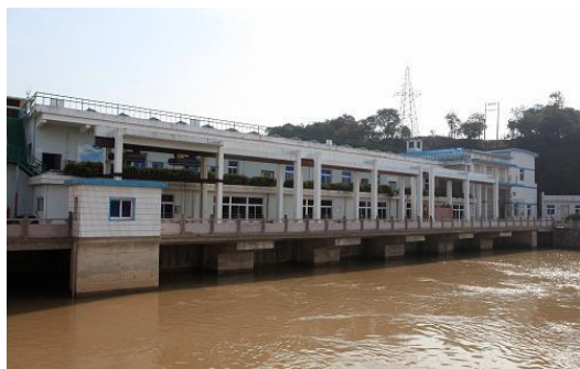
Figure 8. Jiangxia Tidal Power Station
